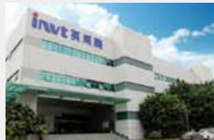
Shenzhen Fuyong Industrial Park
